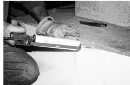
Cut liner around piers leaving approximately six inches and seal with White Seaming Tape to secure. The addition of RadonShield around piers is optional.
