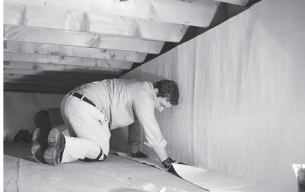
Using the supplied concrete drill bit, drill your first hole (drill hole deep enough to allow pin to insert fully) approx. 2 - 3 inches from the top of the liner and about 6 inches to 1 foot from the foundation corner. Push in Button Fastener (supplied), tap in place with a hammer, if needed. Some diagonal cutting may be necessary at the bottom of the corners to make liner lay flat on floor.
